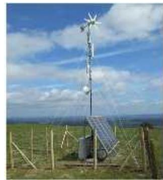
Each of the Ecopops can be powered by a wind turbine, solar panels or both. All of the masts have been thoroughly tested to withstand west coast weather.
