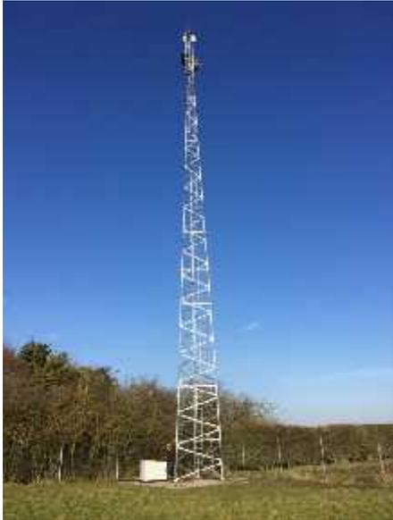
This is an example of a mast that will make up the main ring. Most of the masts will be less than 20 metres tall.
